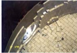
Bricklining work under process
