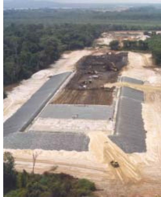
Sealing of landfill (vevy lagoon2)
