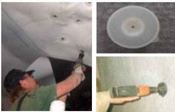
The geotextile is mounted by fixation discs shot into the concrete
