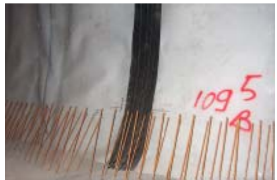
Installation of waterstop profiles at bulkhead sections
