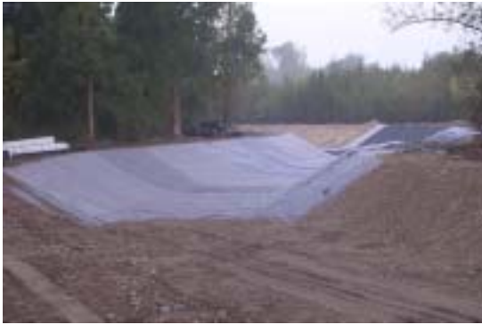
Liner with geotextile protection and backfilling of gravel
