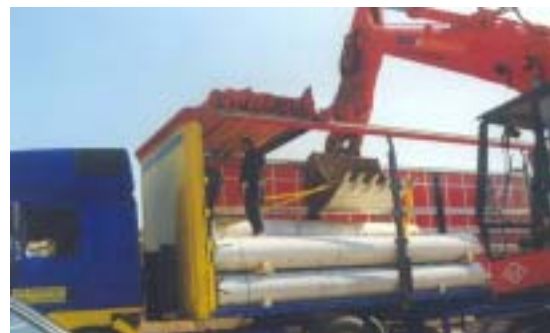
Deloading on site
