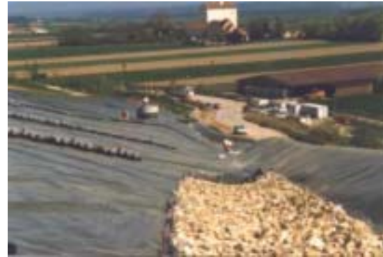
surface drainage at landfill capping
