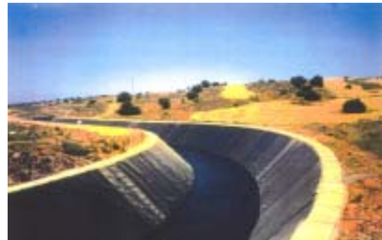
Sealing of water channel (ganez 22)
