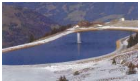
field of application: sealing of waterstorage pond for artificial snow production
