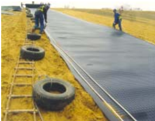
Slope sealing with structured liners
