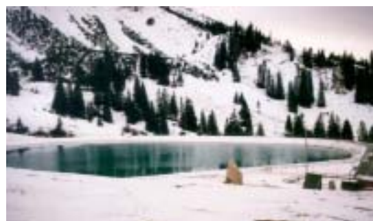
Agru liner under tough condition
