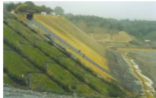
Sealing of extremely steep slopes with AGRU liners.
