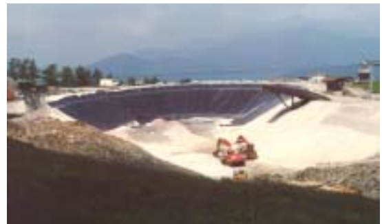
pond in Construction phase
