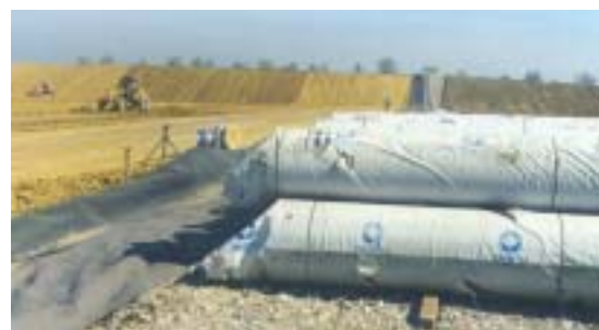
Liner stock on site
