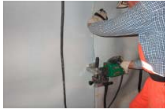
Welding of liners is executed by hot wedge double seam technology
