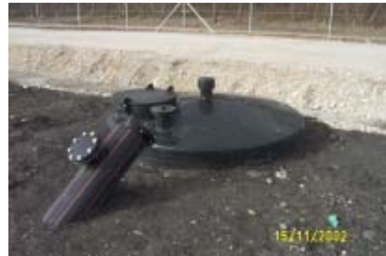
Picture: Gas well collecting system
