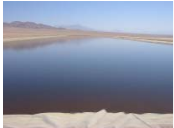
● field of application: waste water settling pond
