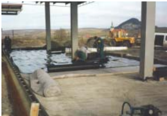
Base sealing of Petrolstation
