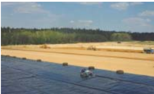
Subsoil preparation for the following day’s lining progress
