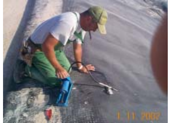
control of the welding seam by air pressure test (Bacci 1602)
