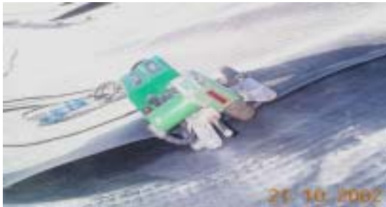
Figure 1 – double track fusion weld (hot wedge weld)
