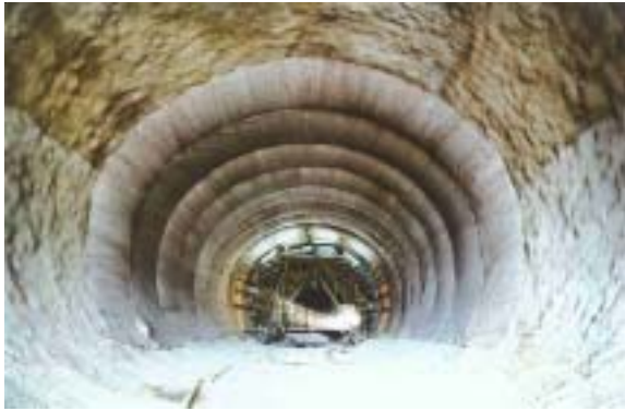
Front: Geotextile, mounted to the shotcrete surface
