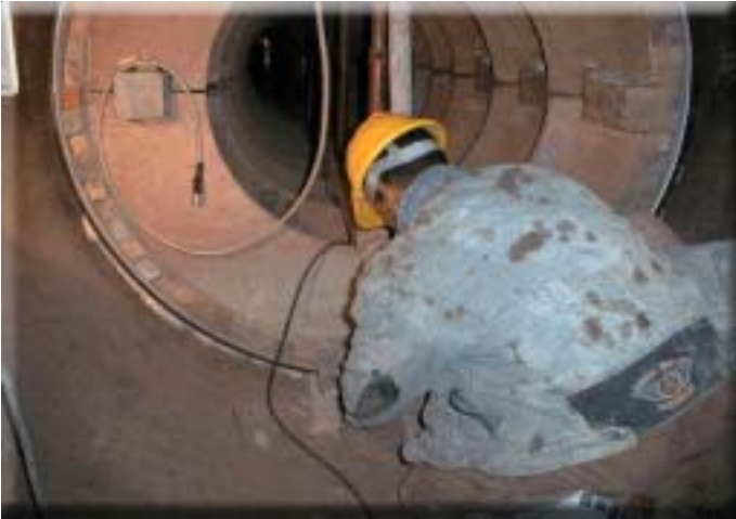
Abbau der Schalung dismanteling of formwork
