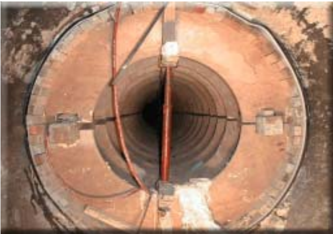
Schalung for dem einfuellen des Moertels formwork section prior to grouting
